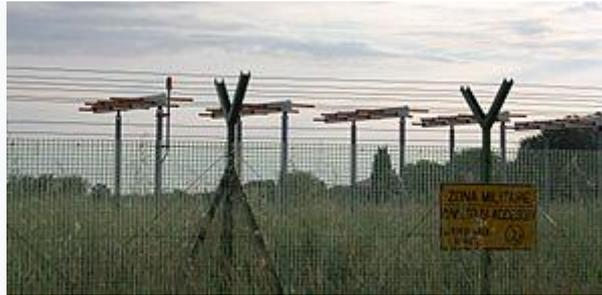
Fig 4.30 Details of five antennas of the ILS at Pisa Airport, Italy
